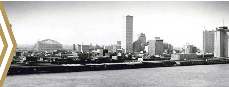
1971 Superdome breaks ground after legislation is passed in 1966 by the largest margin in Louisiana history.
